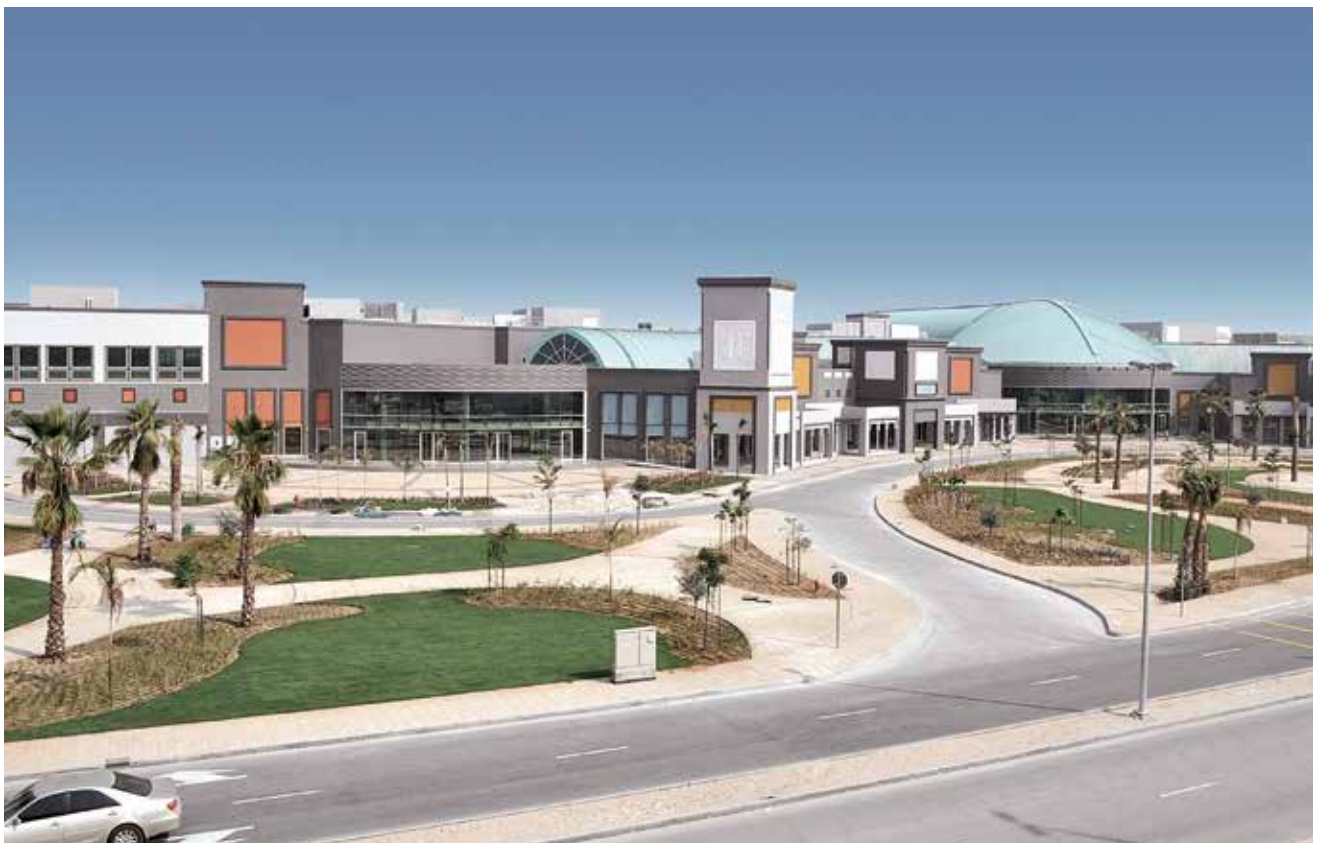
Deira Water Front Market in Dubai Complete equipment of the fish market with 2,000 emergency lights. Back-up is provided by a battery-supported power supply installation.
