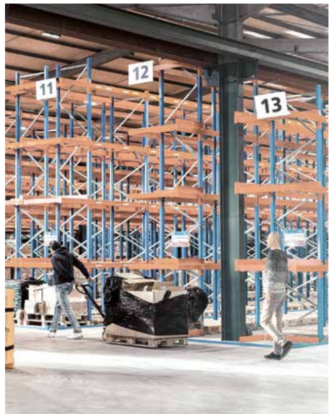
RP-Group warehouse in Rodgau (Germany) Optimum lighting with 90% energy savings: the lighting in the RP-Technik battery warehouse is controlled fully automatically via CASAMBI using a bluetooth connection. This step allowed the energy consumption to be reduced from 12,000 W to just 1,100 W.
