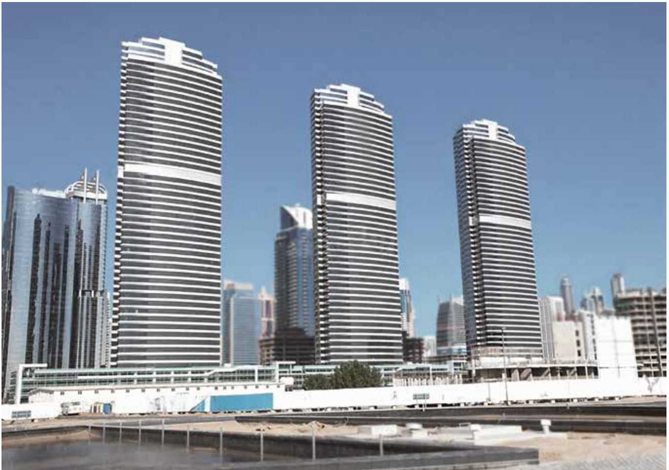
Mazaya Residence in Dubai For ultimate safety: complete equipment with 1,200 emergency lights, secured by a power supply installation with battery back-up.
